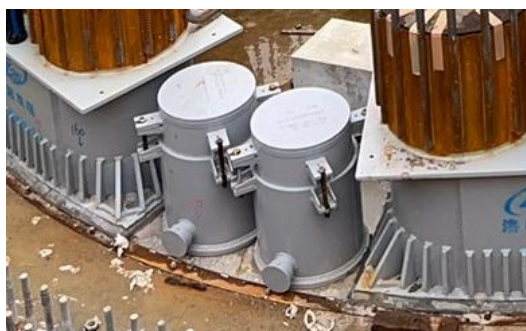
Figure 4.18 - Pre-load of the sandbox
