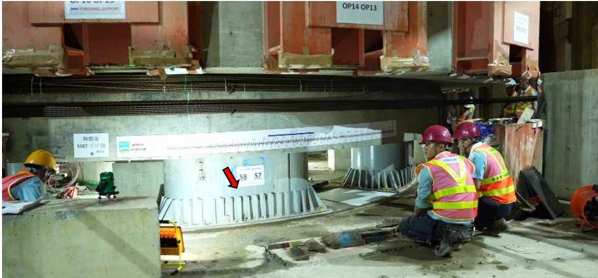
Figure 4.15 - Stanchions before rotation
