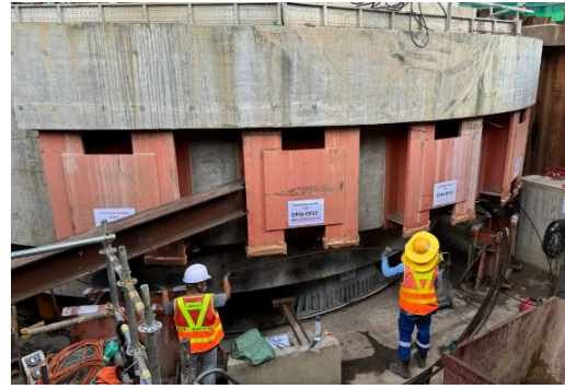
Figure 4.44 - Fixing traction strands
