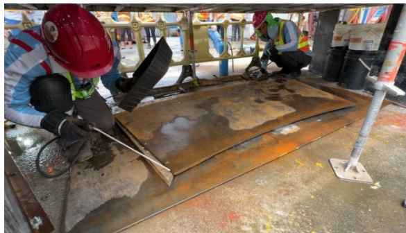
Figure 4.24 - Shimming and Spot Welding at Stanchion
