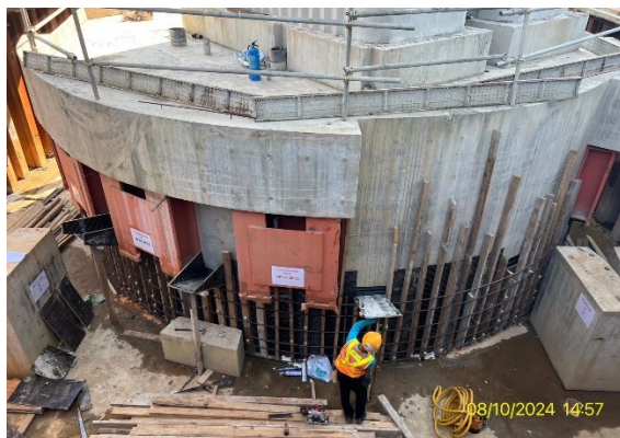
Figure 4.55 - Concreting for Stitch
