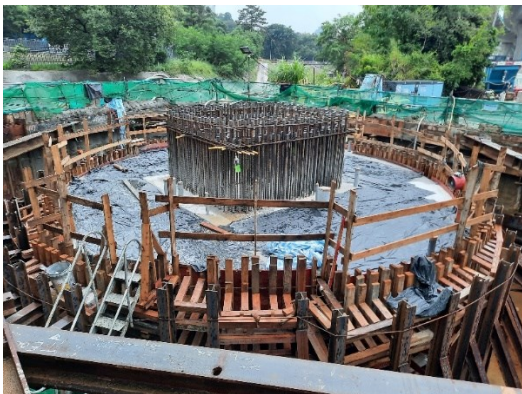
Figure 4.11 - Upper turntable casting
