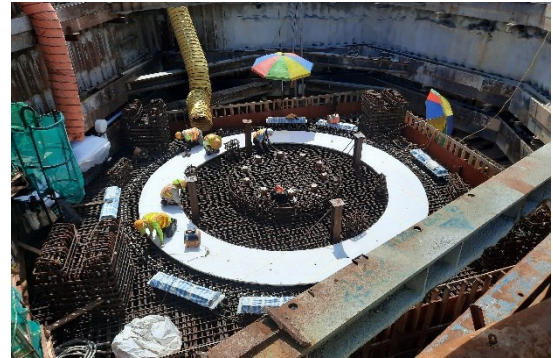
Figure 4.9 - Installation of sliding track
