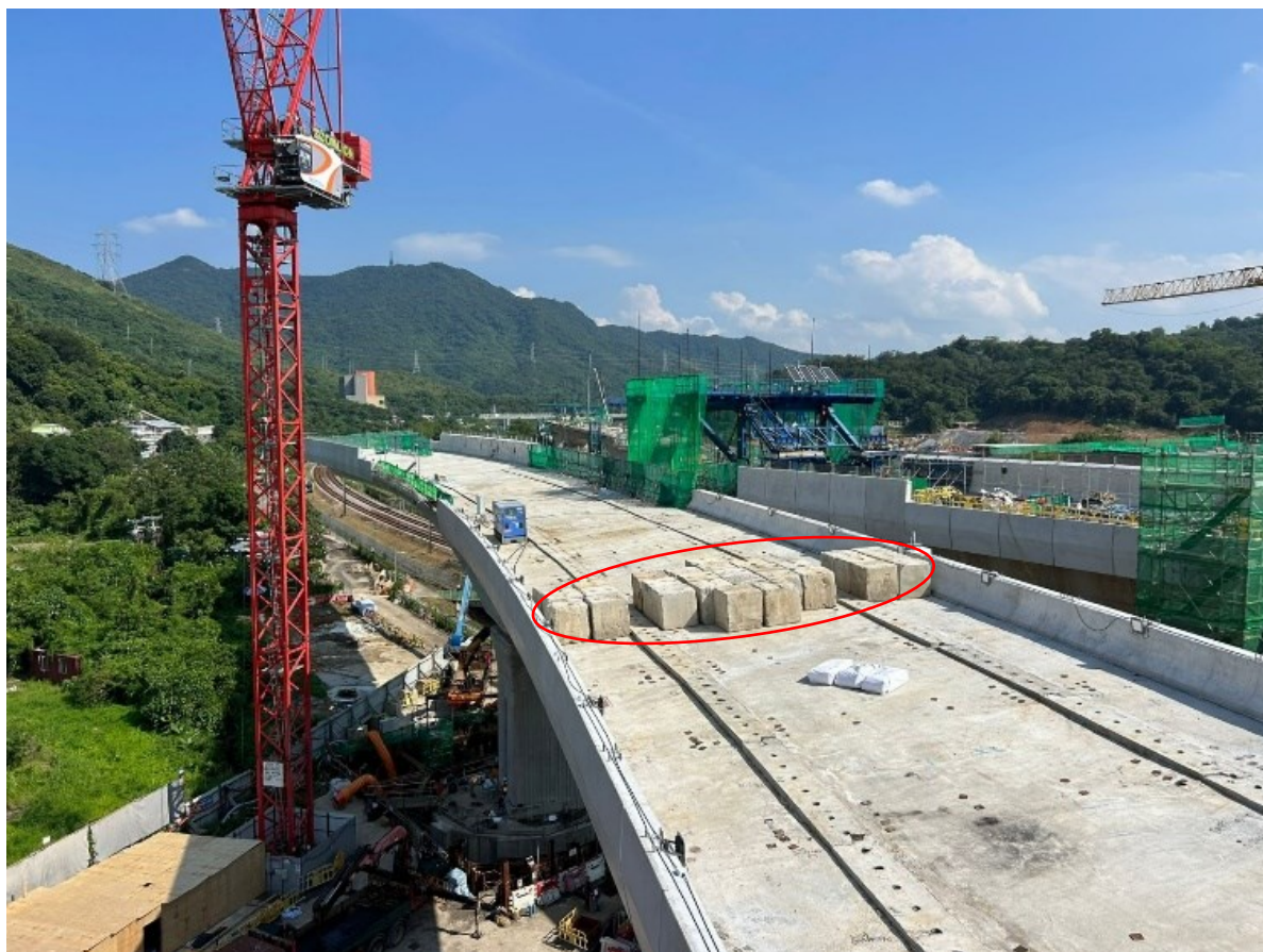
Figure 4.49 - Counterweight Concrete Blocks for Weight Balancing
