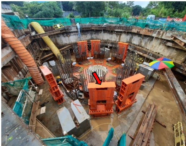
Figure 4.13 - Temporary supports installed on lower turntable prior to the casting of upper turntable
