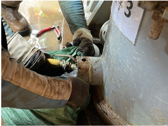
Figure 4.45 - Removing the quartz sand
