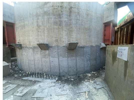
Figure 4.56 - Post-concreting condition of the stitch
