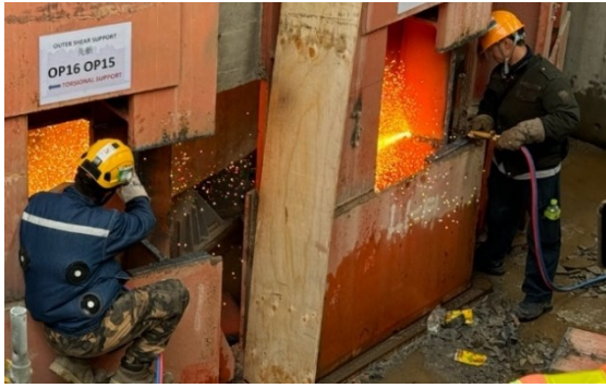
Figure 4.43 - Cutting of shear supports
