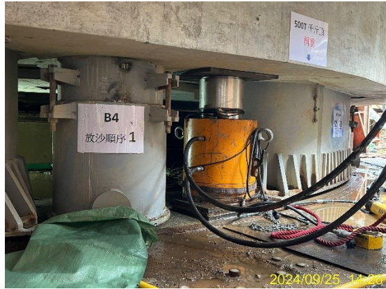
Figure 4.46 - Sandboxes and hydraulic jacks
