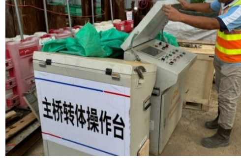
Figure 4.38 - Control station for hydraulic strand jacks
