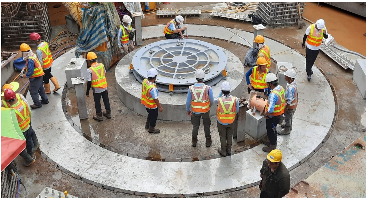
Figure 4.6 - Spherical Bearing Installation
