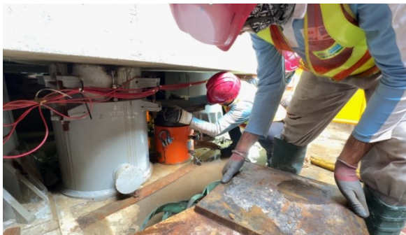
Figure 4.23 - 500 Ton Jack Installation
